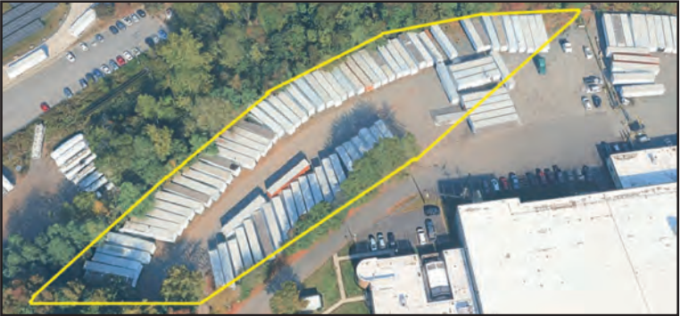
2.2-acre IOS property on Harmich Rd. in South Plainfield
